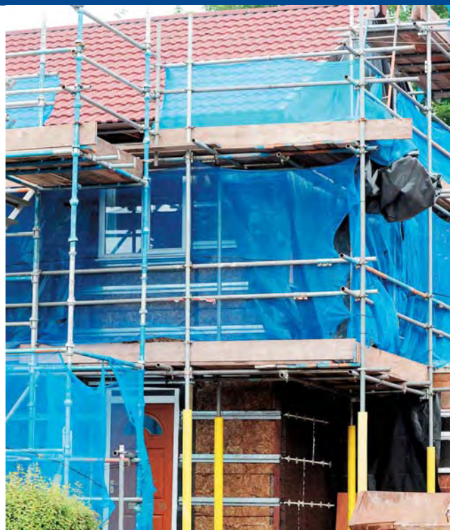
Work to install the cork insulation underway.
